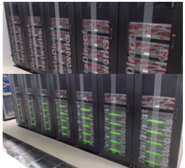
Storage system of Oakforest-PACS
