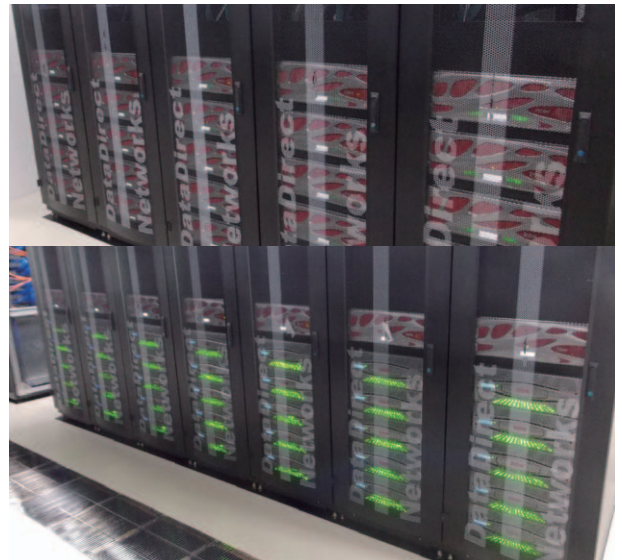
Storage system of Oakforest-PACS
